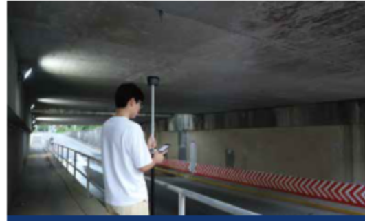
ROAD CONSTRUCTION SURVEYING
